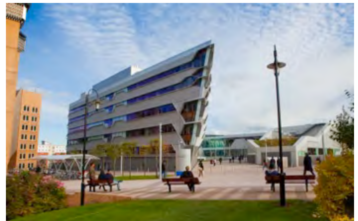
Coventry University's Engineering and Computing Building
