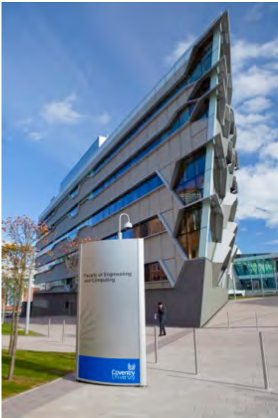
Coventry University's Engineering and Computing Building
